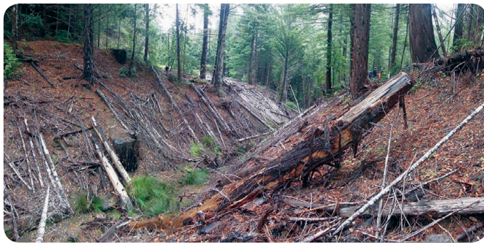
This shows a very large haul road crossing removal and daylighting of more than 100 yards of Steelhead habitat that was buried by aggraded material behind the haul road stream crossing. We're talking about 10,000 cubic yards or more removed and trucked to a stable flat at some distance away. The burying of and/or blockage of Steelhead habitat was a common occurrence during the tractor logging from 1946 and even into the early 1980s. For scale, note the people in the upper right.
